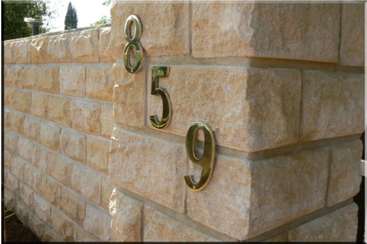
Corner Bonding Details 15.01.1/2 Series 150 Cottage & Executive Range
